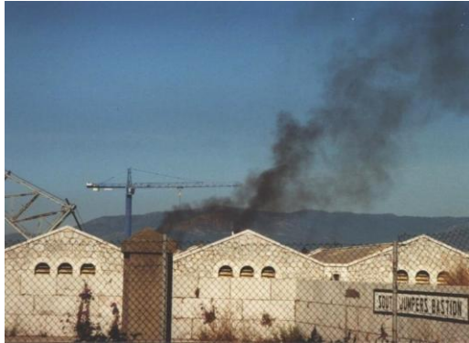
OESCO Power Station Poorly applied technology
